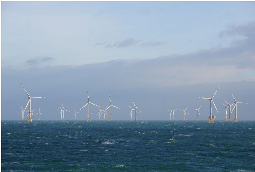
Offshore wind farm. © Fraunhofer IWES/Gerrit Wolken-Möhlmann
