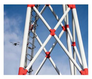
A drone being used to inspect an offshore wind turbine. © Fraunhofer IFAM | Picture in color and printing quality: www.fraunhofer.de/en/press
