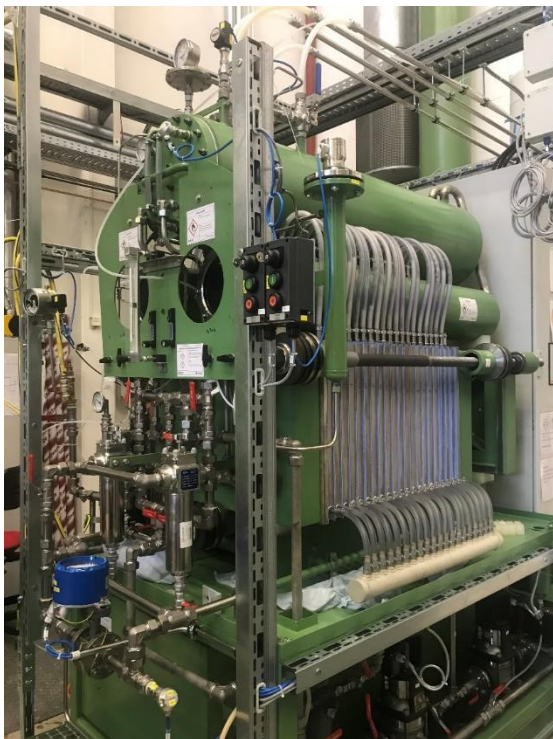
Industrial alkaline atmospheric test electrolyser at Fraunhofer IFAM Dresden
